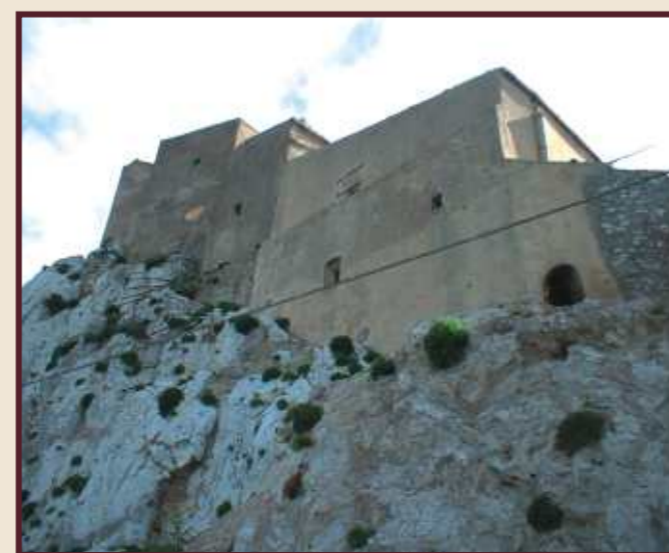
4. Ellipsactynia fossiliferous limestones, interbedded with silicious argillites and radiolarites acting, in this case, as foundation for the building of hystorical residential areas of Sclafani Bagni.
